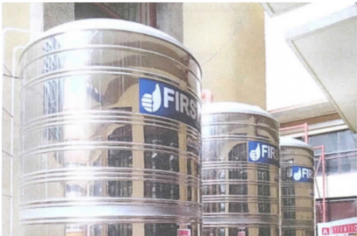
Rainwater Storage System at the Diego Silang Building
