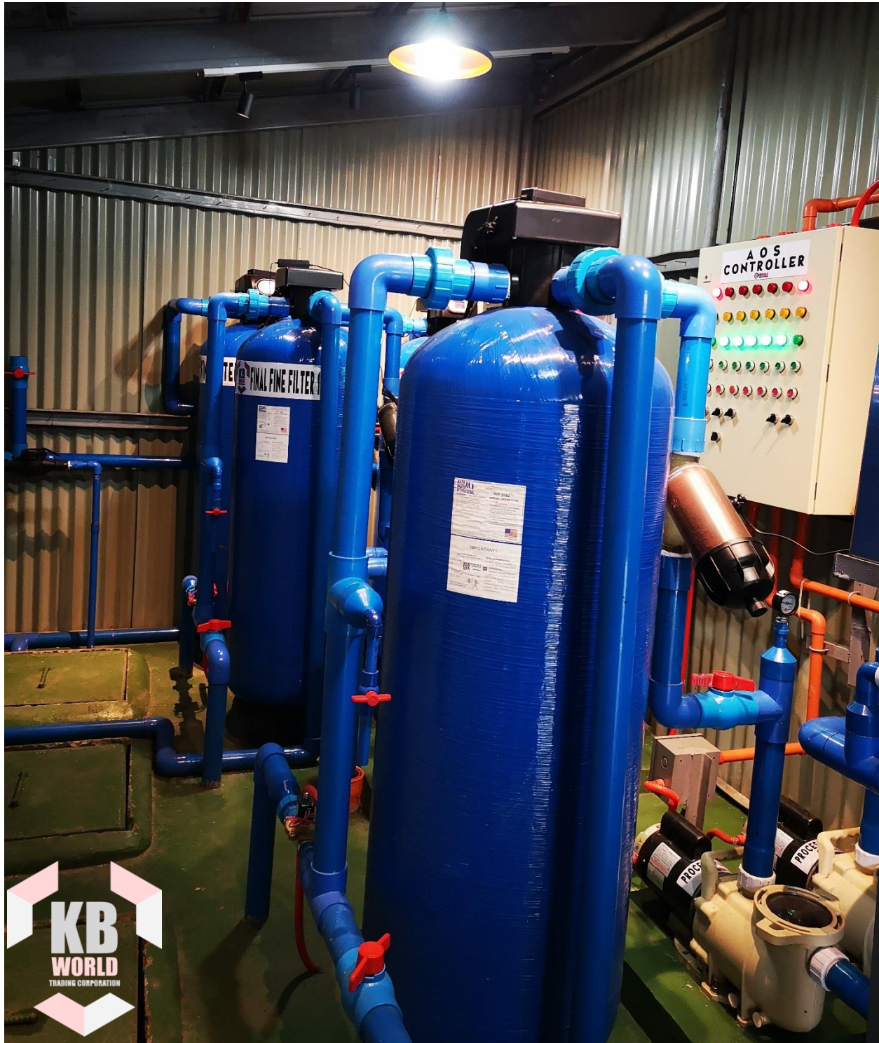
PHOTO INSIDE THE FACILITY SHOWING FINAL FINE FILTERS
