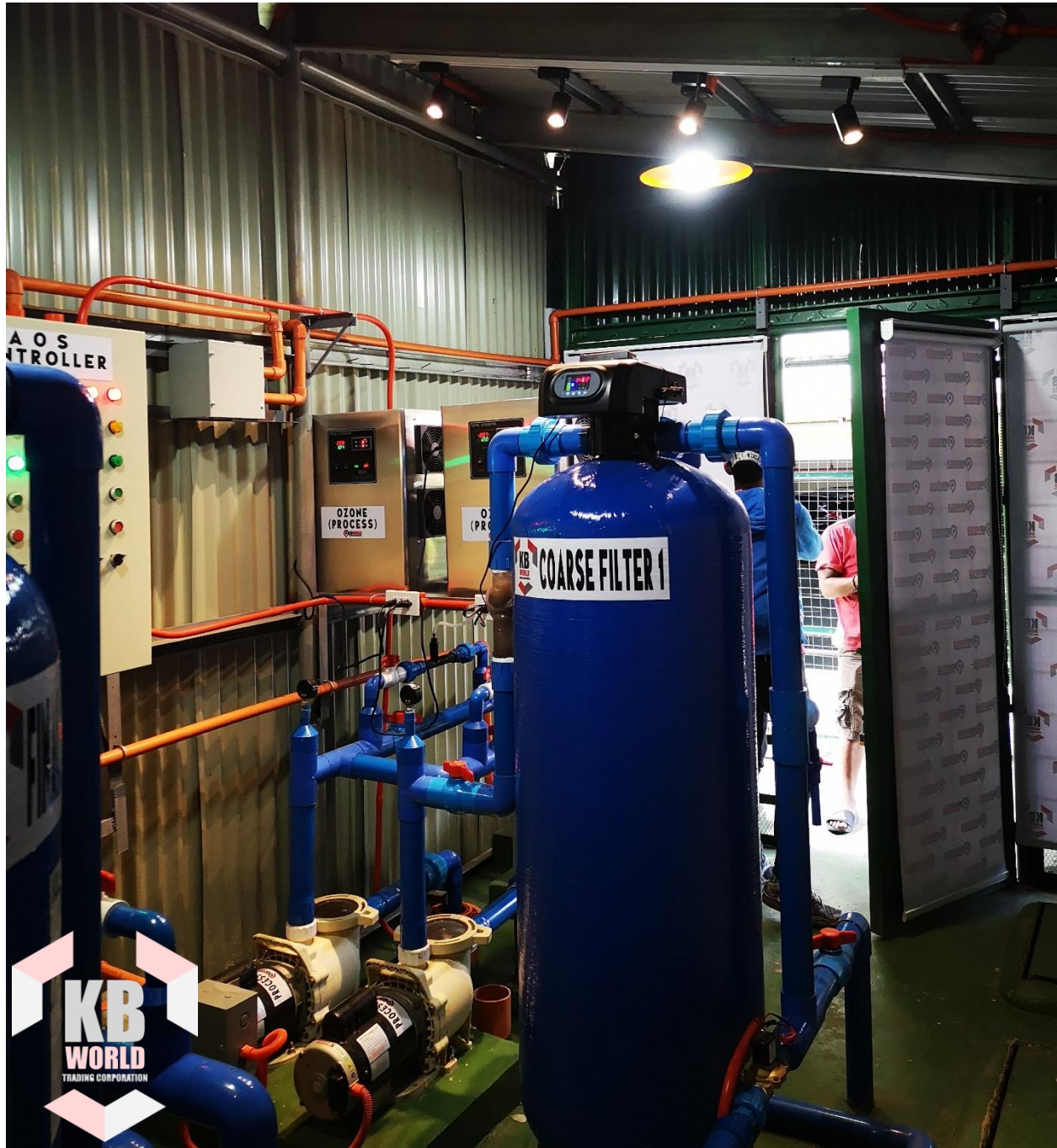
PHOTO INSIDE THE FACILITY SHOWING COARSE FILTER AND OZONATION UNITS
