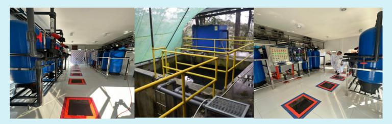
In partnership with KBWorld Trading Corp. and Hyper Kem and Machineries, Inc., SLU has implemented advanced wastewater treatment systems at both the Main Campus and Mary Heights Campus. These systems use ozonation and biofiltration to eliminate contaminants while preserving essential minerals, ensuring treated water is safe for reuse.
